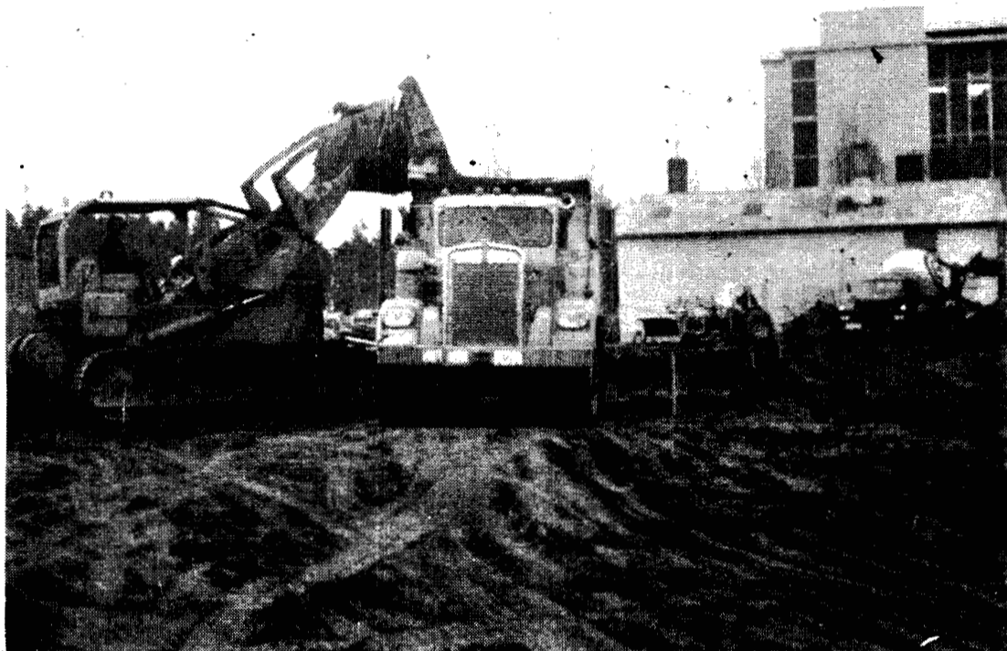
The powers that be have escalated their war against the environment. It's the new extension to the Clearihue Building to give the students more classrooms and the faculty more offices. I guess we'll have to find a new site for the annual kite festival.
